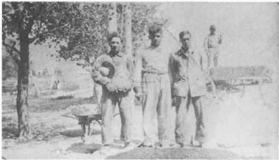
Constructing a sidewalk at Iosepa about 1910. (Utah State Historical Society)
