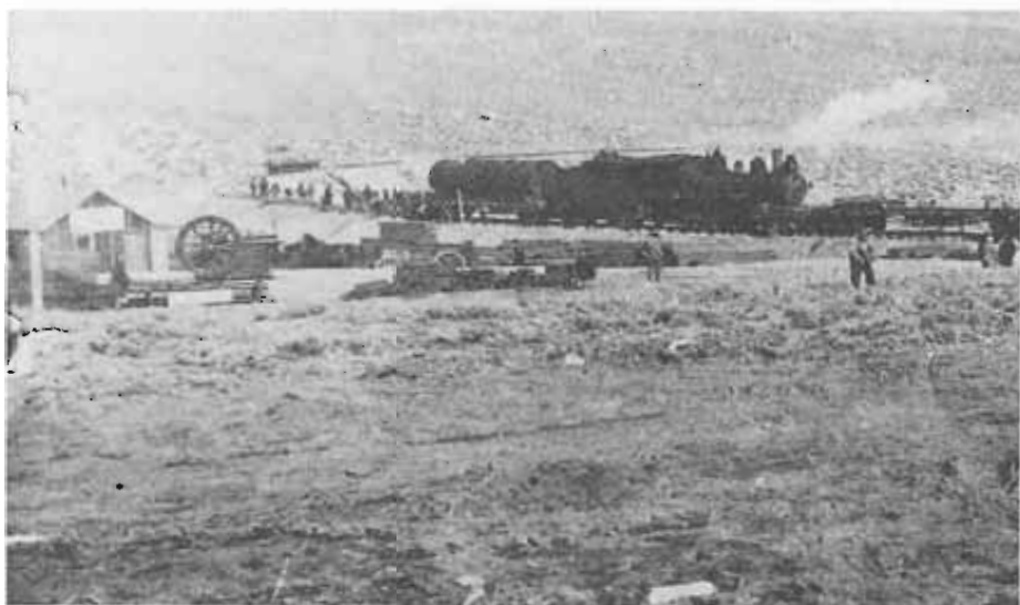
Laying track for the Deep Creek Railroad at Gold Hill in 1917. (Utah State Historical Society)
