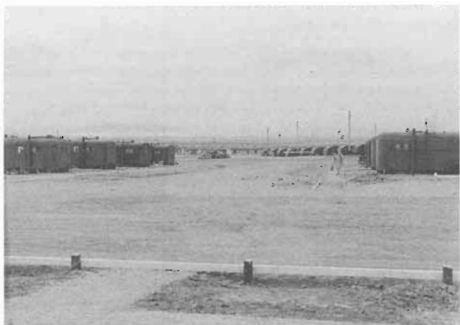
Trailers were used as temporary housing for International Smelting and Refinery Company at Tooele. (Utah State Historical Society)
